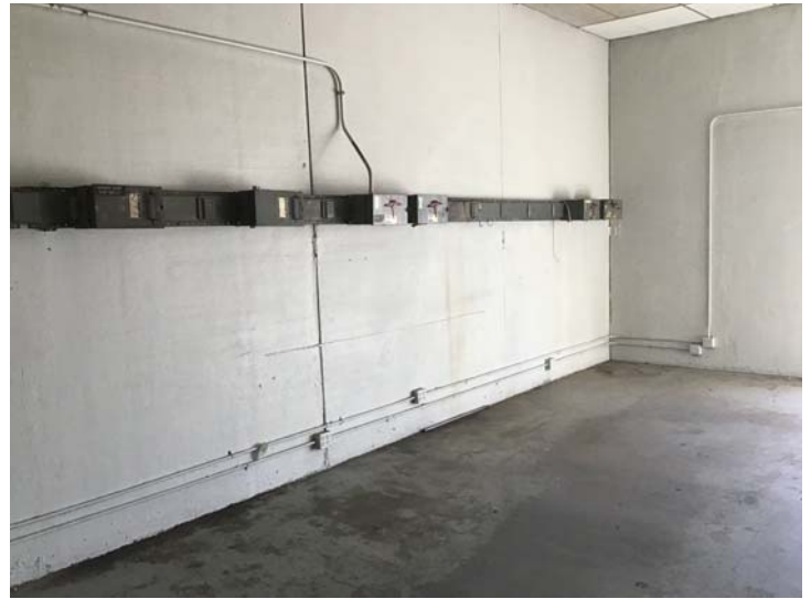
Heavy power installed.
